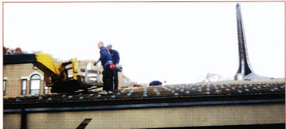
Preparing the tile for shipment to the Pfister stock yard. Photo Courtesy of Pfister Industries, Inc.
