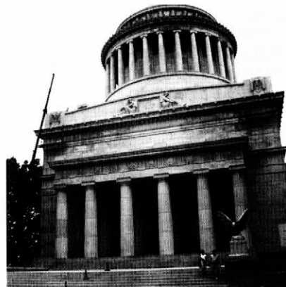
Grant's Tomb during Pfister's roof restoration.
